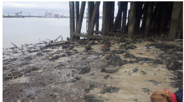
Figure 2.2: Piles under Bell Wharf
